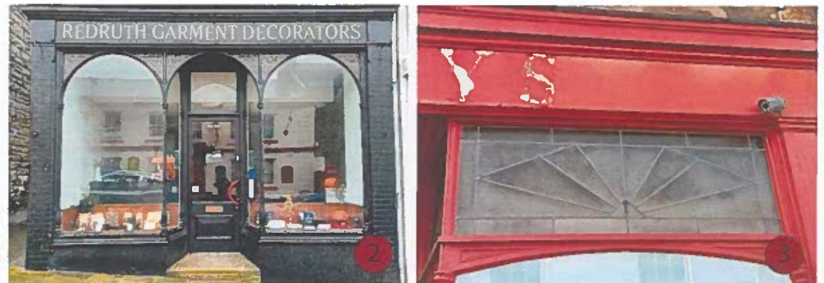
Redruth Drapery Stores, East End. These incised, gilded letters were originally covered by a sheet of reverse painted glass. @ Historic England, James Davies 2021
