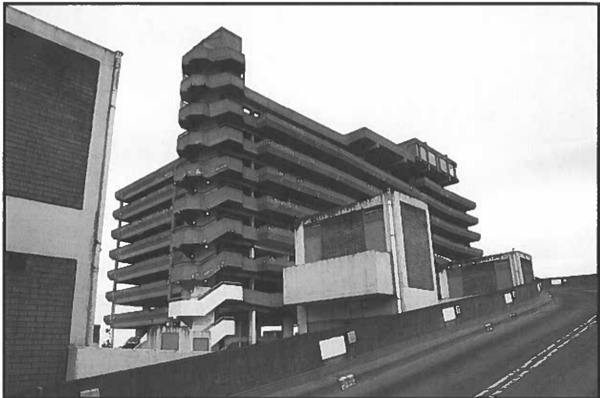
Trinity Square Car Park - now demolished
