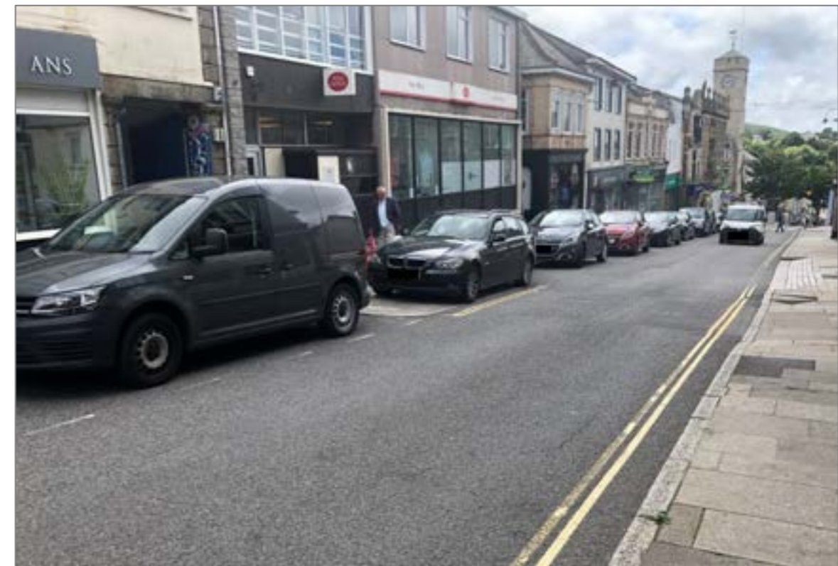
Figure 2.2: Fore Street On-Street Parking Bays – Vehicle using Kerb Build-Out as Parking Space
