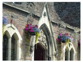
Work has been completed to the boundary walls of St Rumons Gardens with the skilled masons from Regan Builders removing the vegetation, securing the loose masonry and sealing the tops of the walls with a lime render. Now that the area is safe for users and passers-by our next aim will be to improve the look of the gardens themselves with more colourful, wildlife friendly planting schemes.
