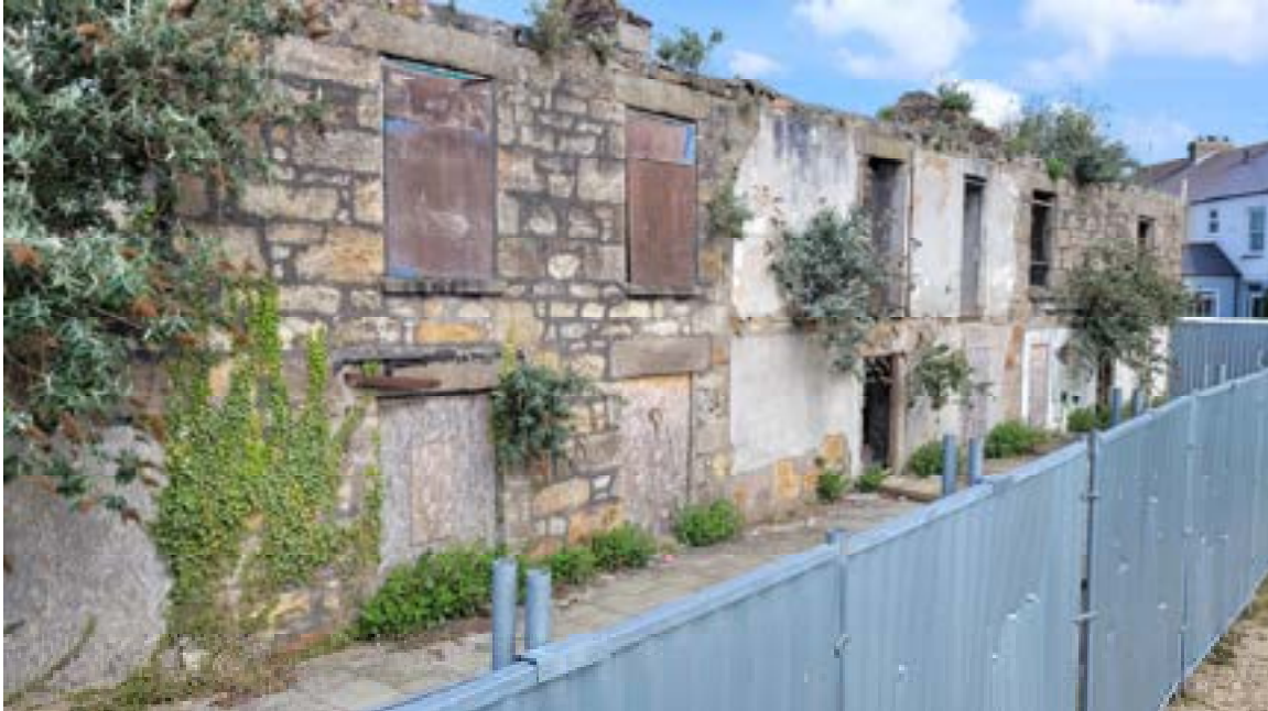
8. East elevation View 2.
