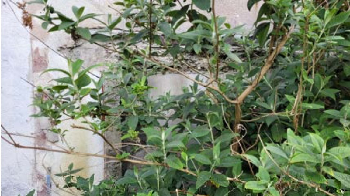
18. Concrete slab cut back to face of elevation. Possibly during demolition of the other buildings on the site.
