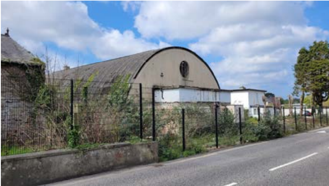
7. East elevation obscured by vegetation.
