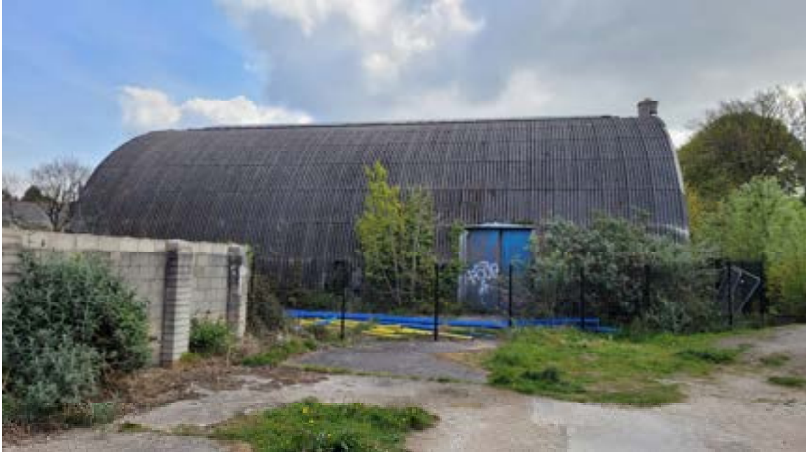
24. West elevation overview.
