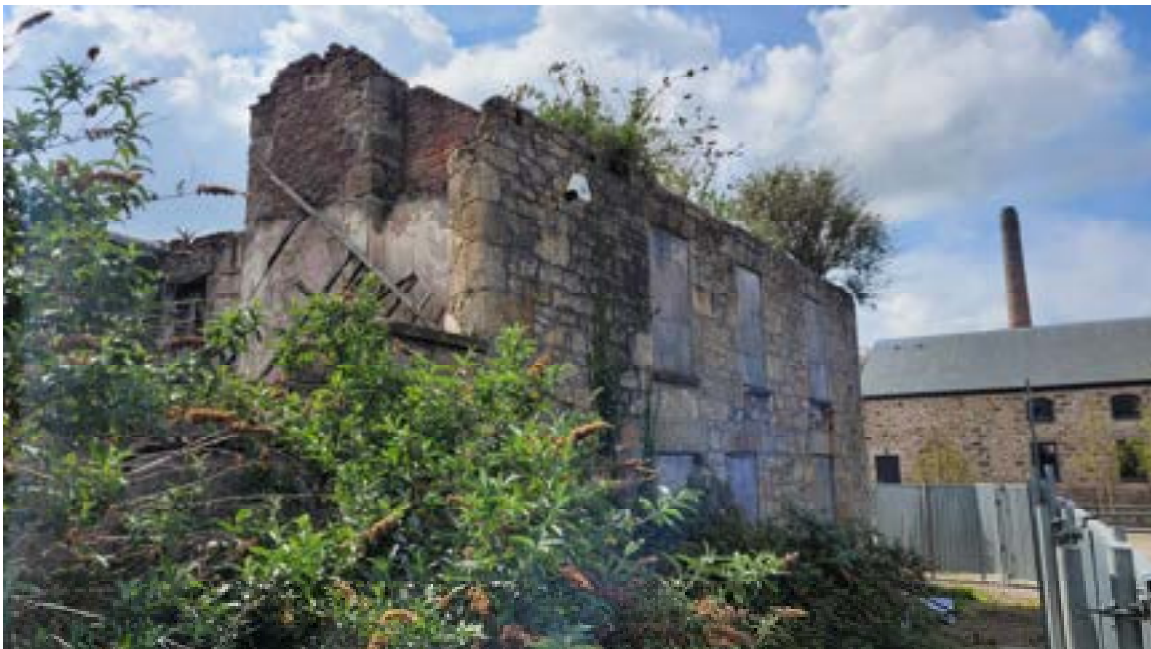
24. Southern end of west elevation.
