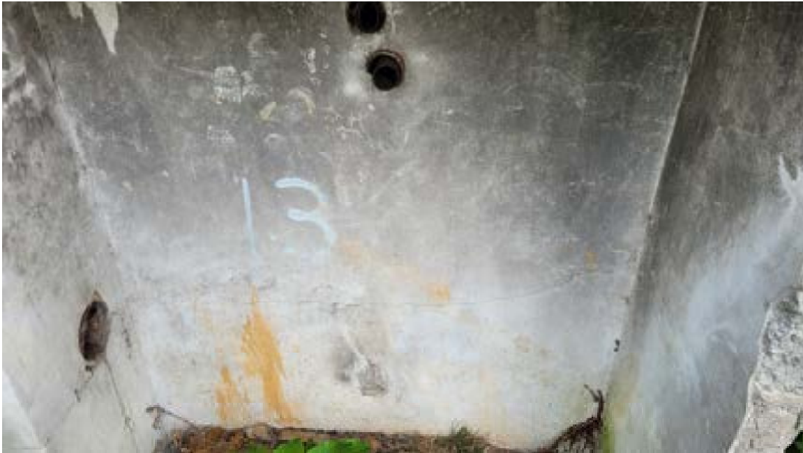
17. Minor horizontal cracking to render to right hand side of chimney on south elevation.
