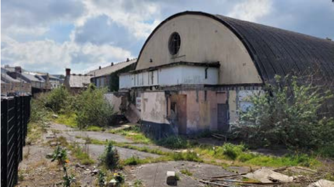
2. Partially demolished cavity wall in foreground.
