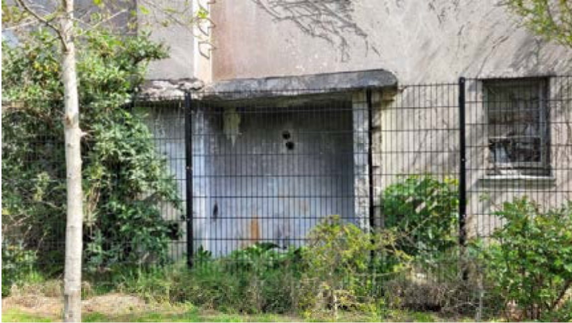
13. Concrete roof slab adjacent to chimney.
