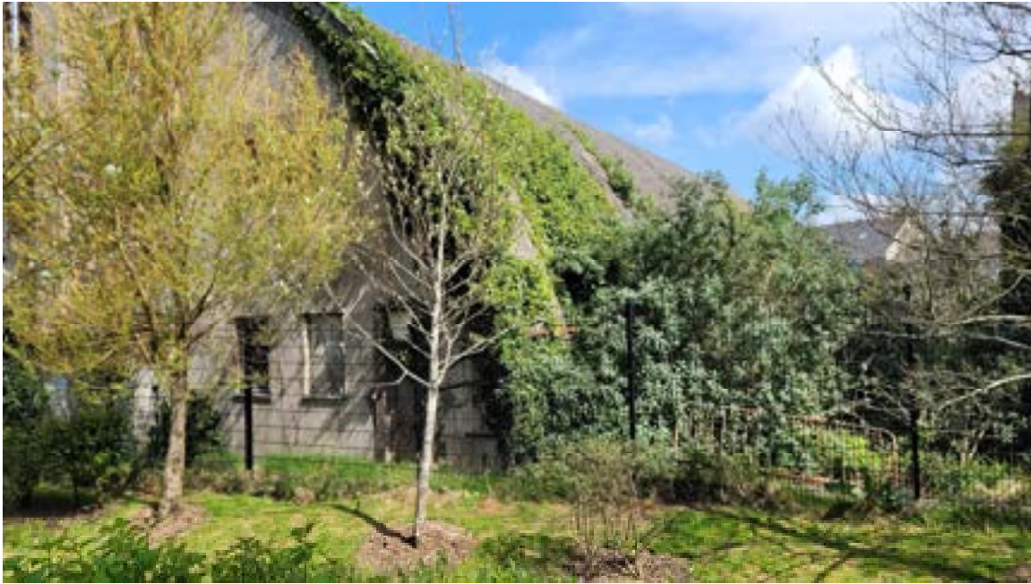
9. East elevation – significant vegetation restricted visual inspection.
