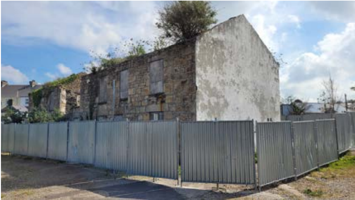
17. South elevation (right of frame).
