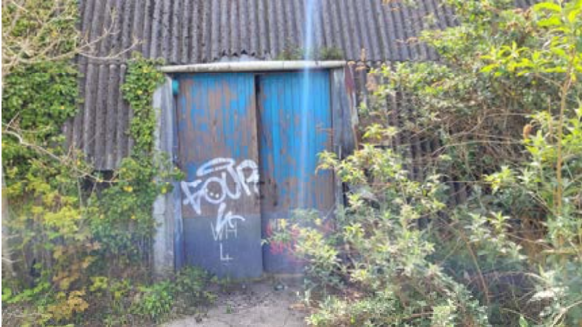
26. West elevation access door.
