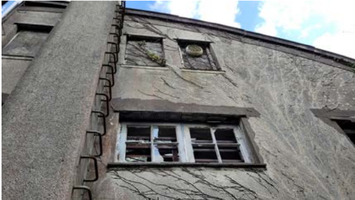
15. Metal ladder rungs embedded into chimney.
