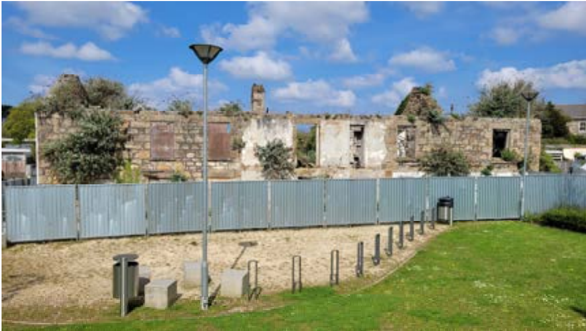
7. East elevation View 1.
