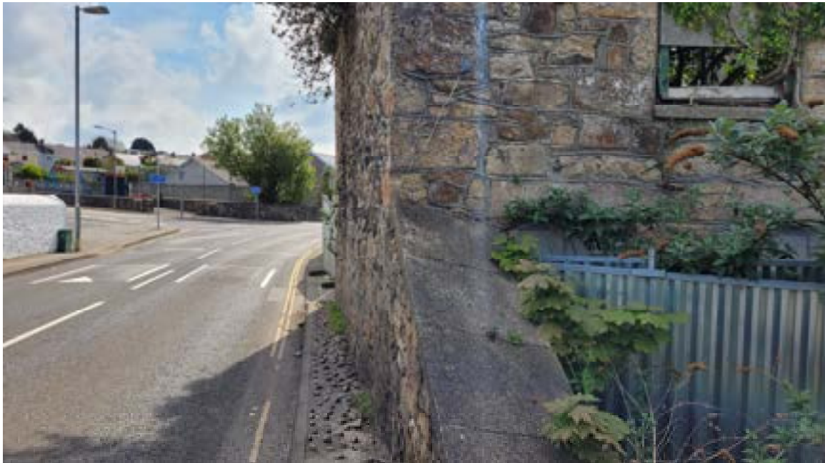
2. Angled concrete coping on boundary wall extending from north west corner of building.
