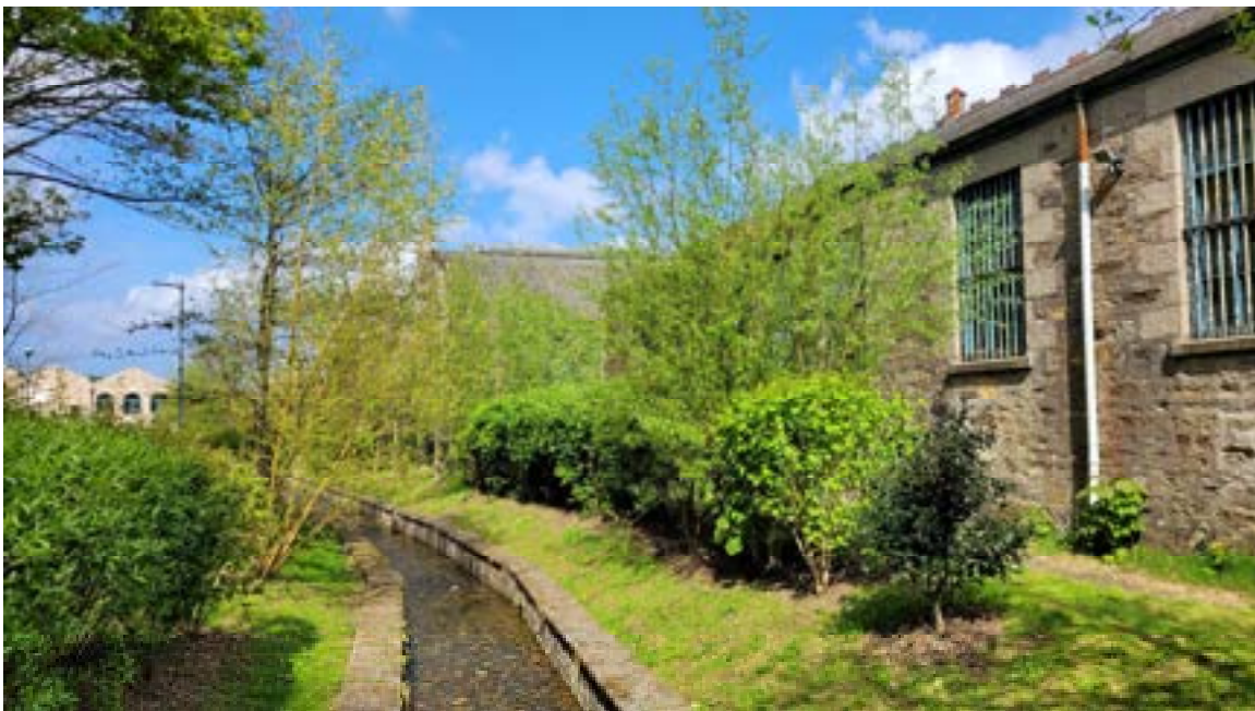
8. East elevation in background showing damage to roof lights to top of barrel vault roof.
