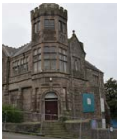
01. The Ladder, Clinton Rd
