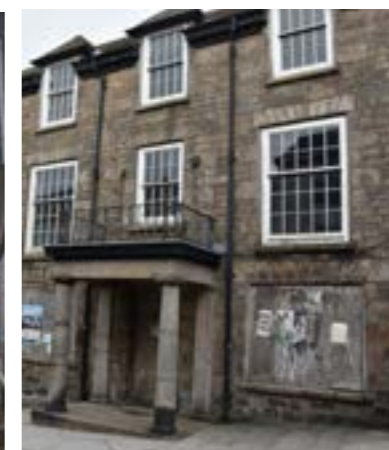
06. London Inn, Upper Fore Street
