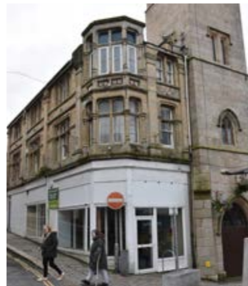
06. 73, Fore St - Former Cornwall Hospice Care
