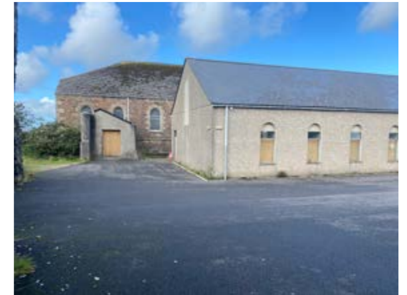
02. External rear of Redruth Methodist Church / Wesleyan Building
