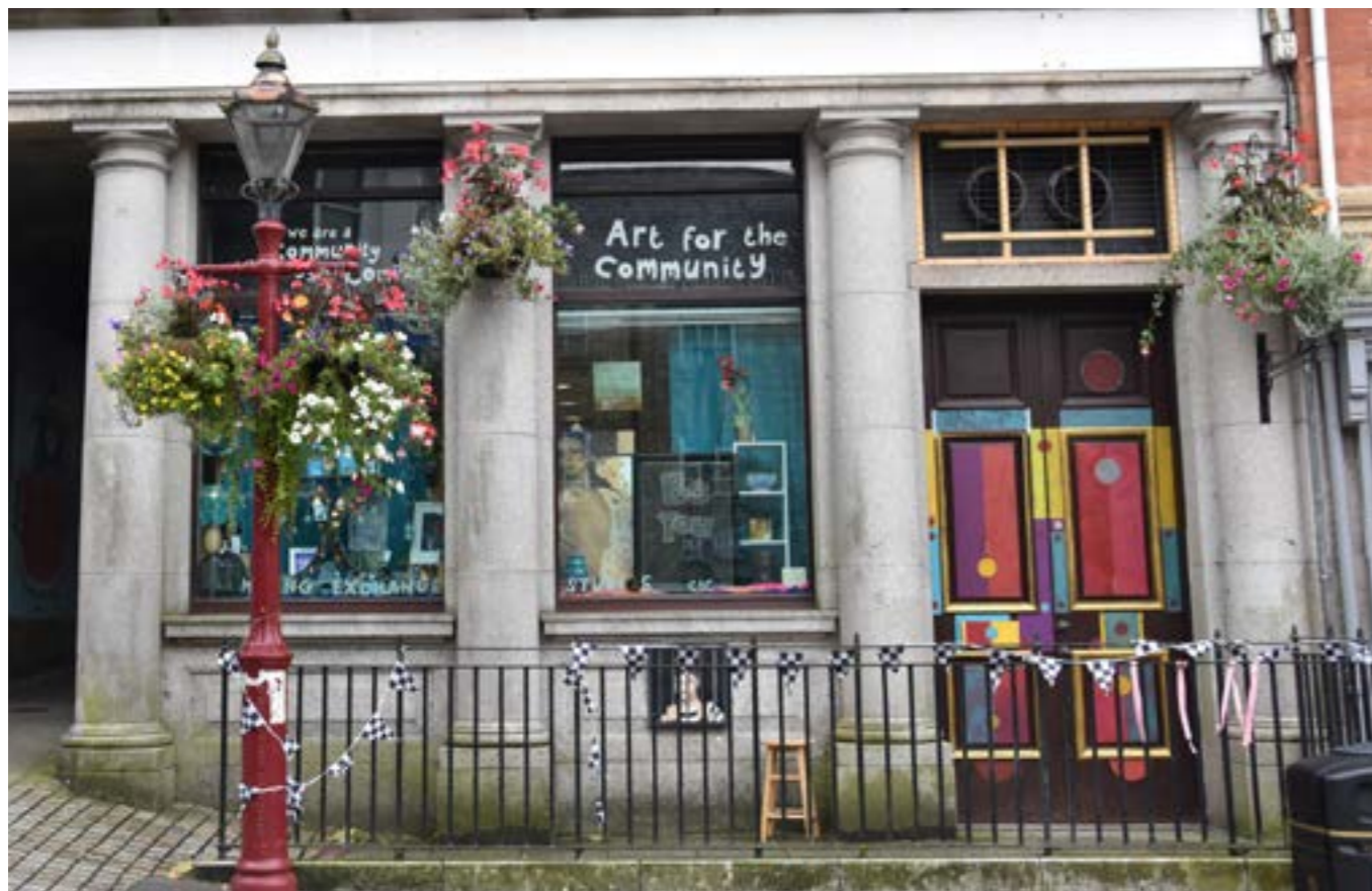
FIG. 035 81, Fore St - Mining Exchange Studios Gallery (Former HSBC Bank)
