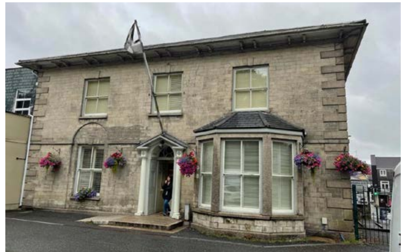
FIG. 036 St. Rumons Club - sash window replacement
