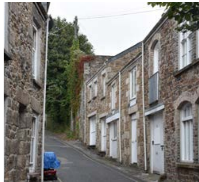
Back Lane West (south)
