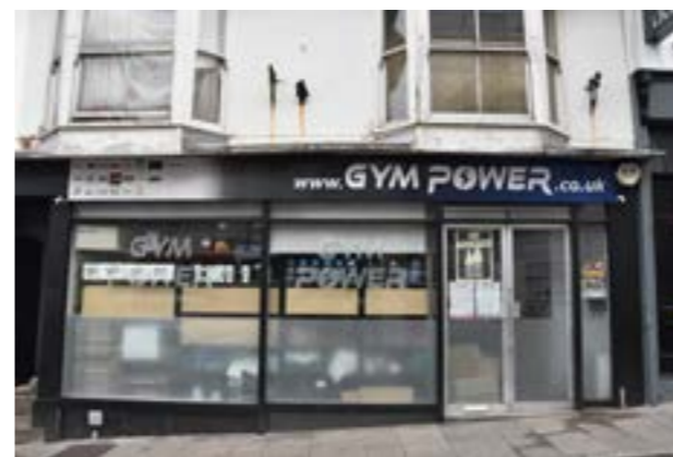
15. 38, Fore St - Gym Power
