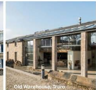
Old Warehouse, Truro
