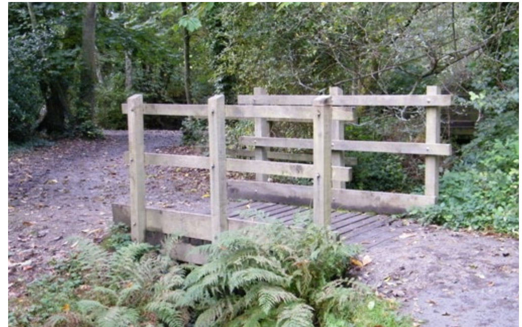
Footbridge over stream, Tehidy Woods, Camborne
